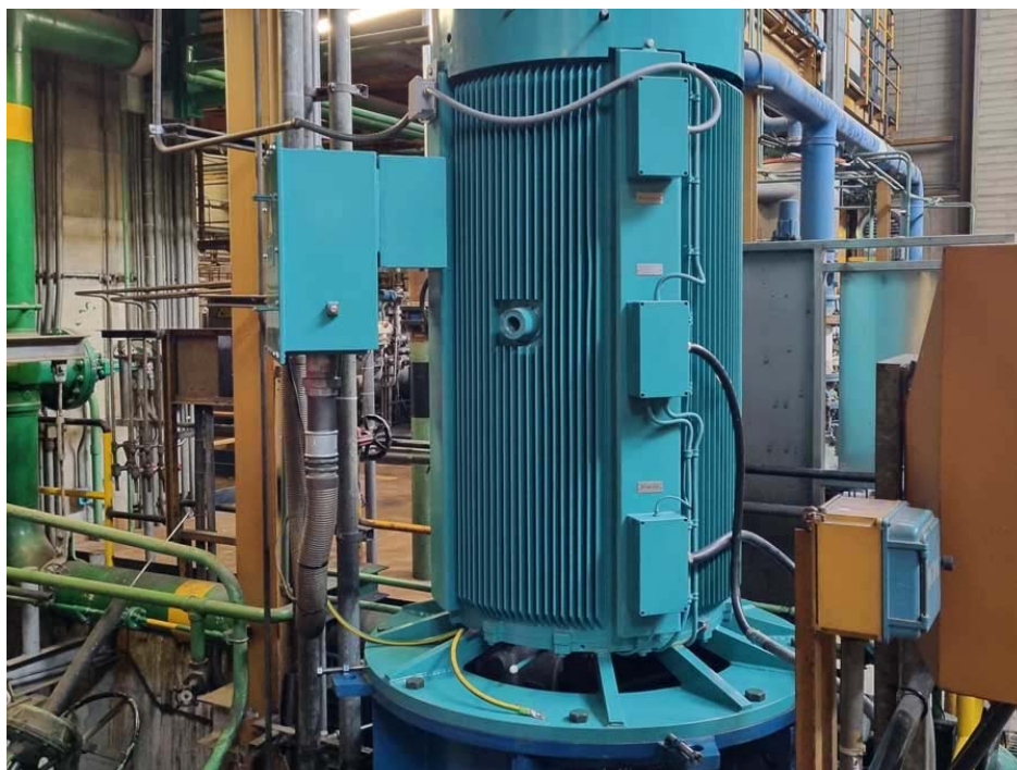
Caption: Menzel adapted the pump motor for the application – with a special flange and repositioned main terminal box
